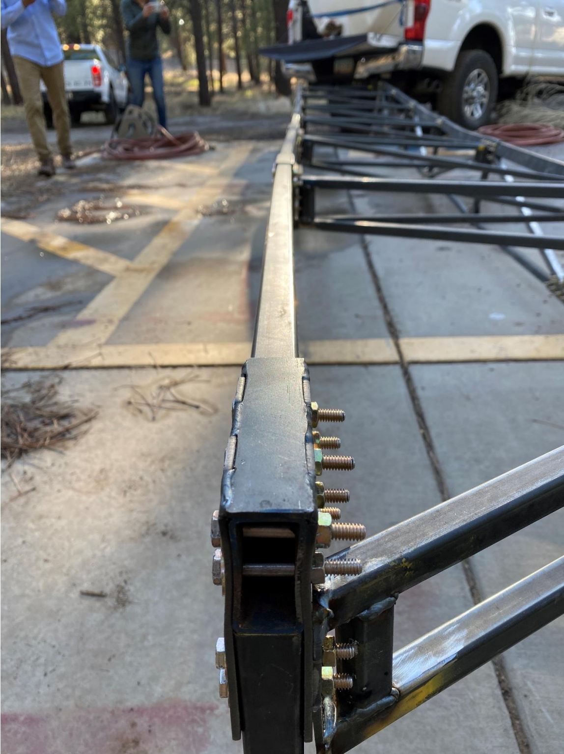
Figure 7: Top chord deformation from loading to failure.
