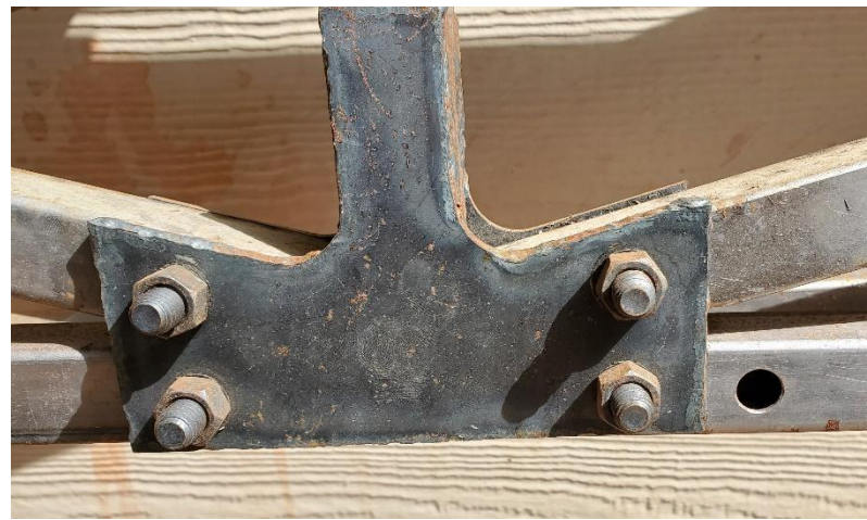
Figure 3: Existing Connection E Conditions
