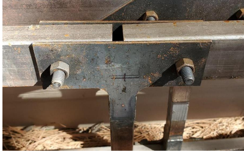
Figure 2: Existing Connection B Conditions
